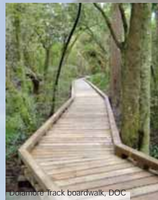
Dolamore Track boardwalk, DOC
